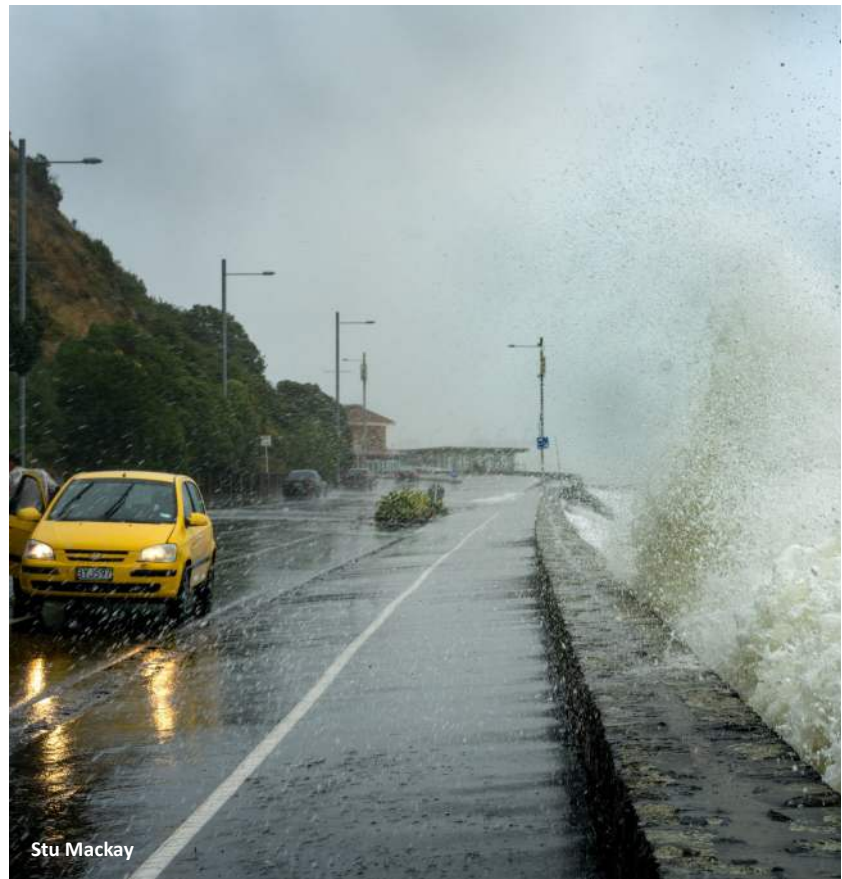
Figure 1. Waves overtopping the seawall along Tamaki Drive, Auckland.
