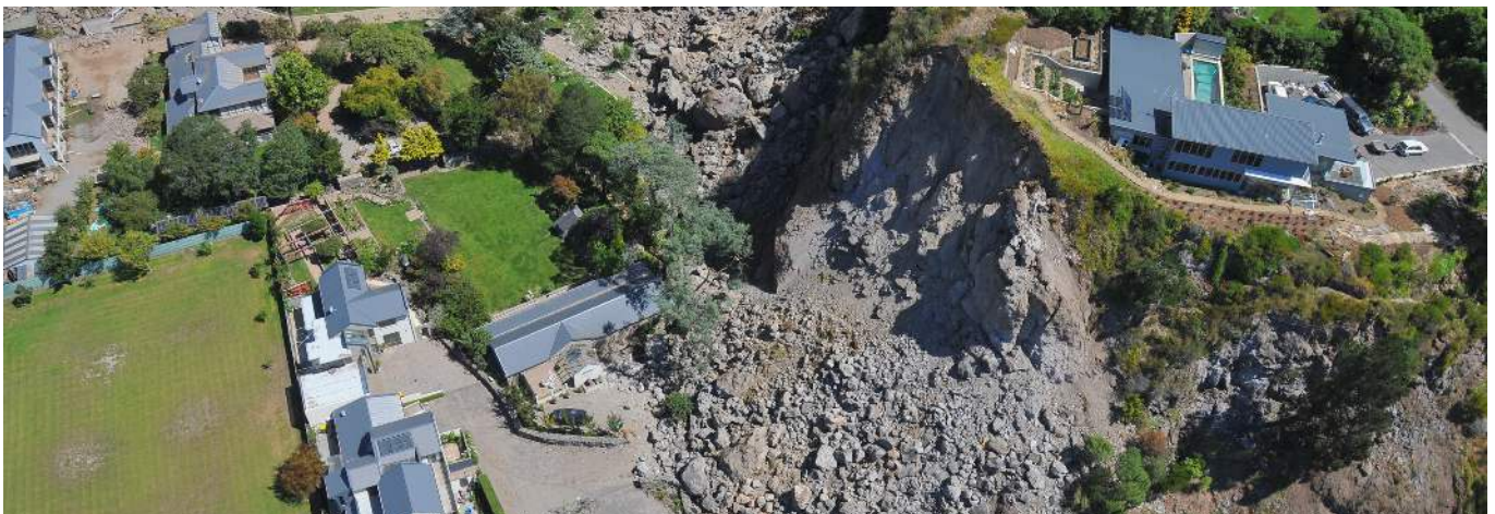
Rockfall damage at Redcliffs following the 2011 Christchurch earthquake. Credit: Graham Hancox, GNS Science | EQC Toka Tū Ake
