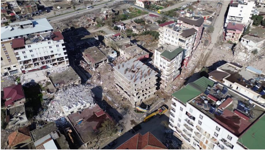
Damage after 2023 Turkey EQs
