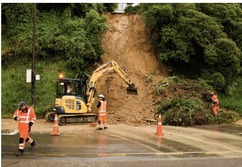
Crews clean up landslips. Credit: Dave Allen, NIWA.
